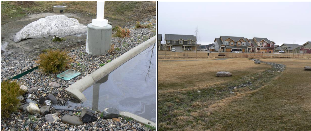
Figure 8-1. Stormwater BMPs: Parking lot designed to drain into a swale and a mixed use development.
